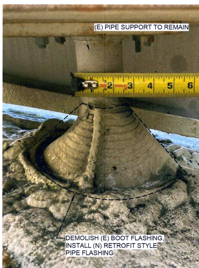
11 A4.1 NTS SUPPORT THRU ROOF
