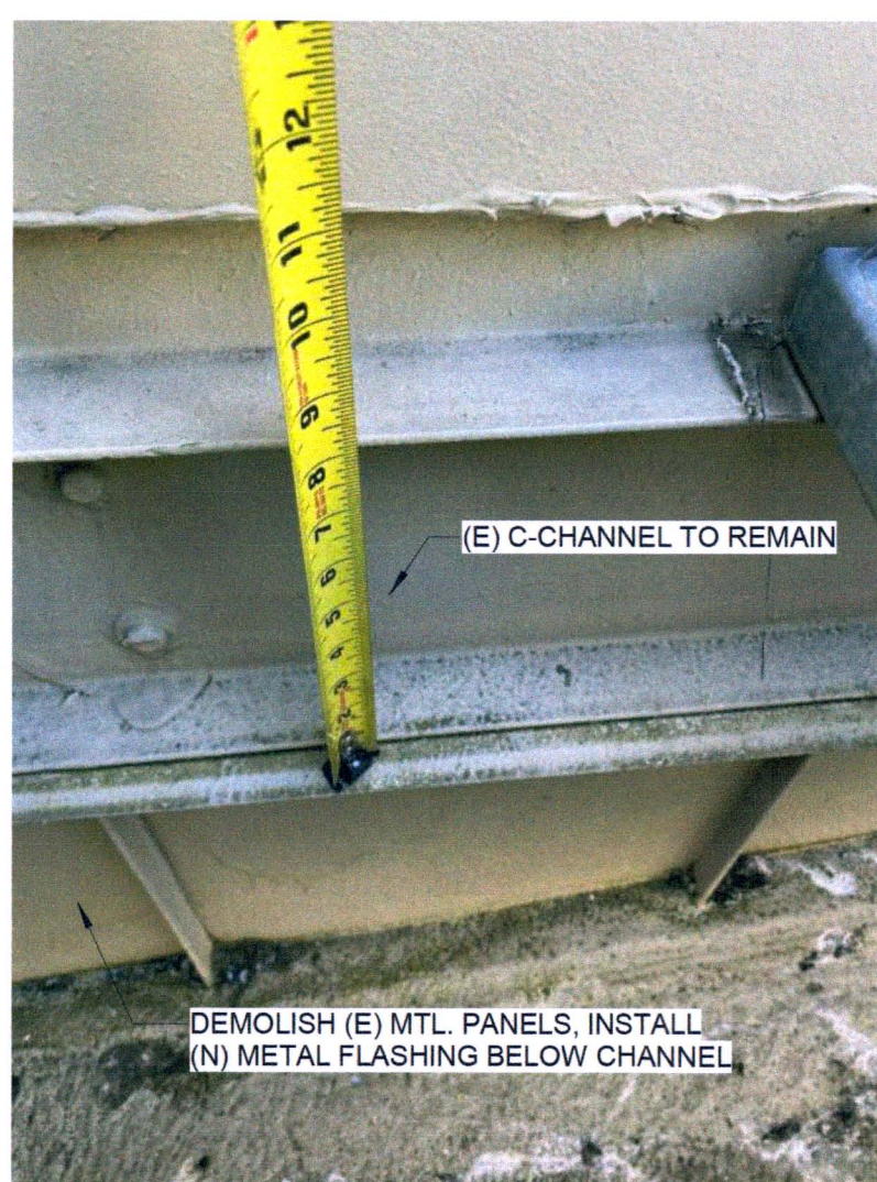
10 A4.1 NTS CHANNEL AT WALL
