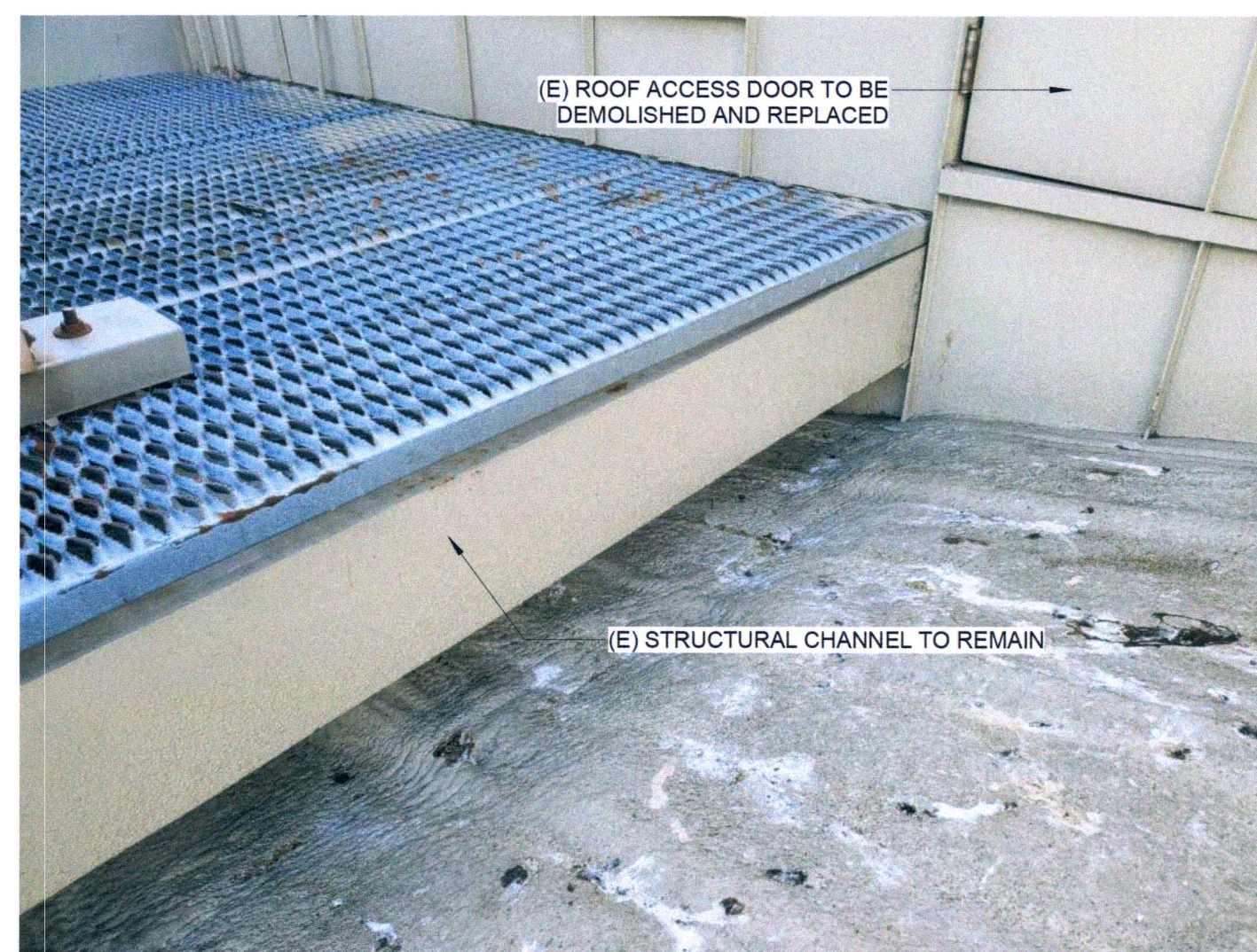
6 A4.1 NTS PLATFORM AT WALL
